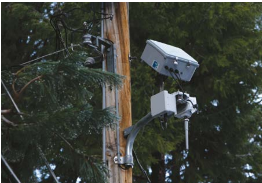
BGAN terminal in a NEMA enclosure, mounted on a remote power pole to backhaul smart meter data collected through an adjacent concentrator and access point.
